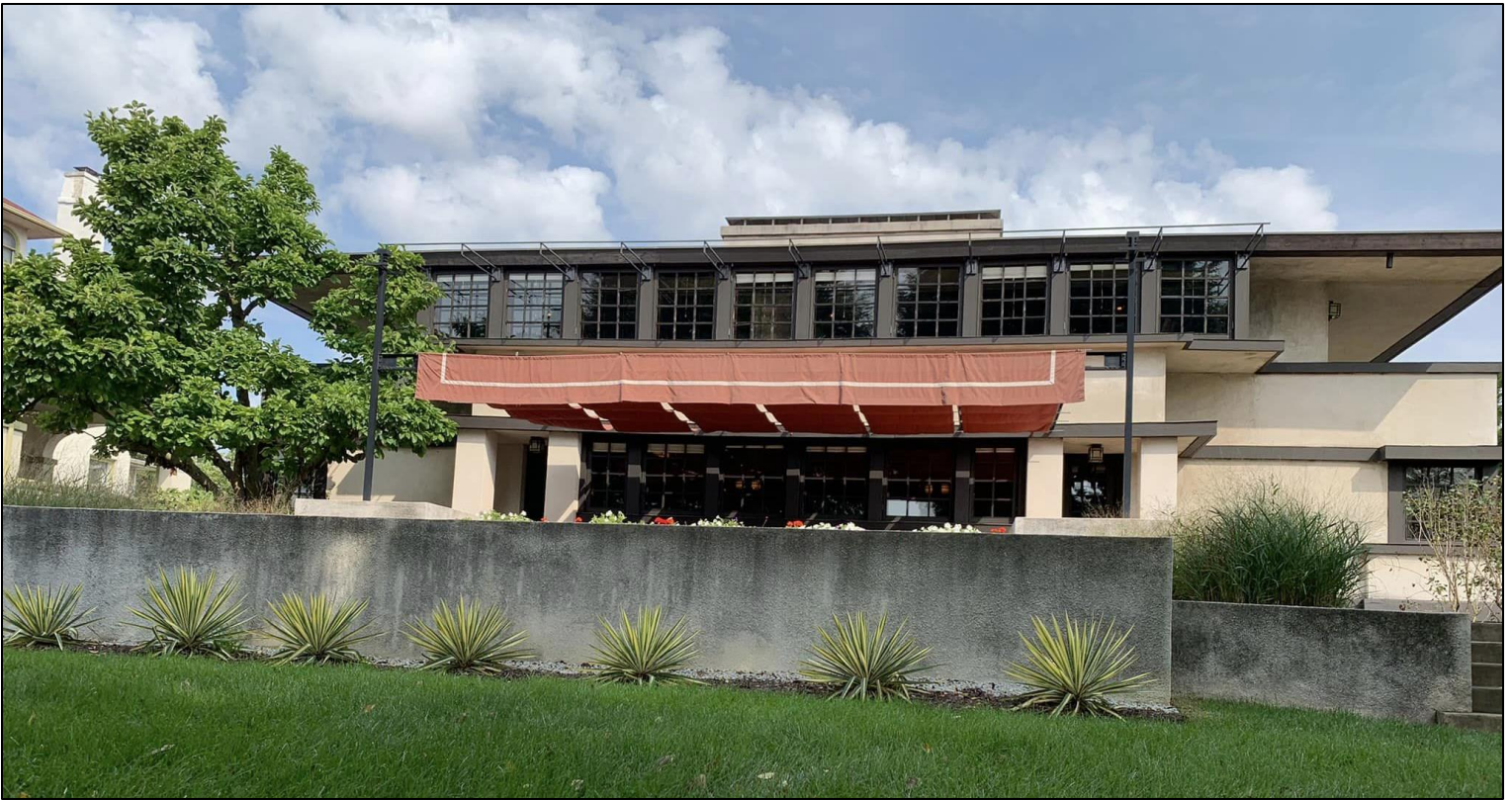
An outside view of Frank Lloyd Wright's Wescott House, located in Springfield, Ohio.
