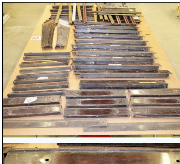
Interior trim being prepared for wood graining.
